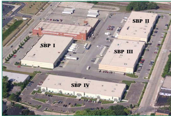
Stadium Business Park
